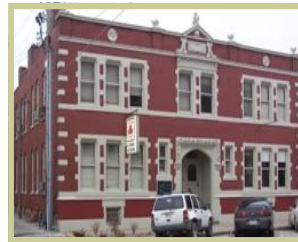
Grim Building 113 E. Washington St.
