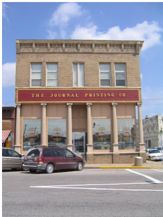
Existing Journal Printing building
