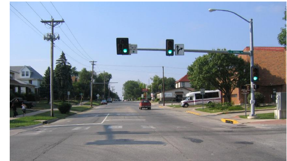
Existing Franklin St. looking North
