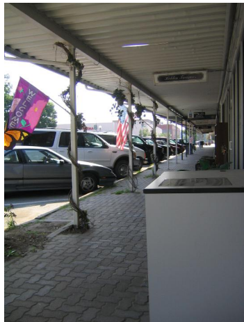
Existing sidewalk canopy
