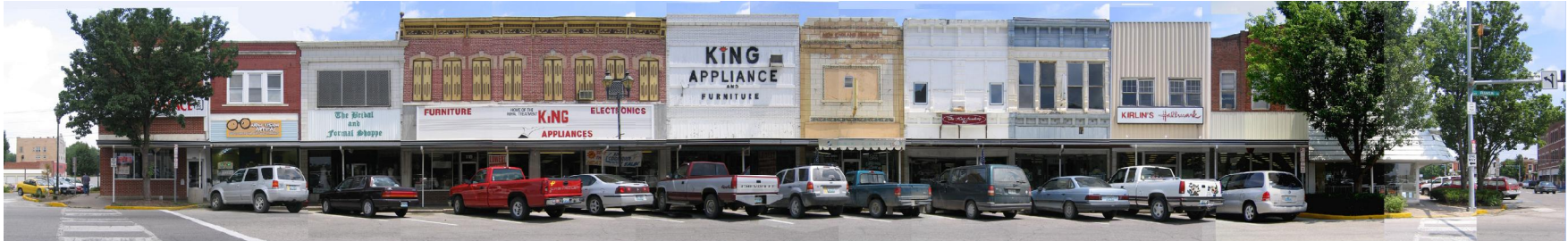
Existing Franklin Street at courthouse square
