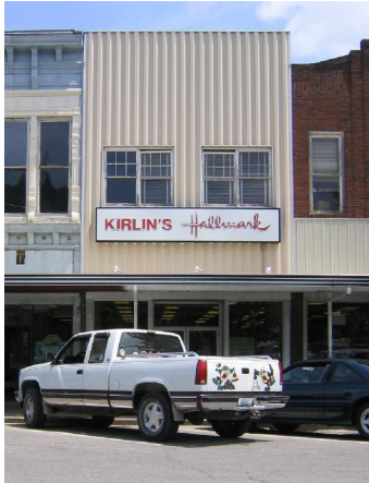
Existing façade covered by metal siding
