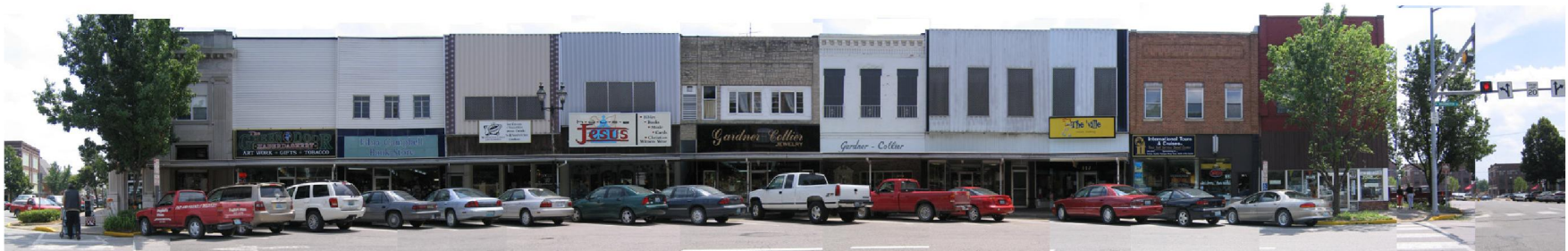
Existing Washington Street at courthouse square
