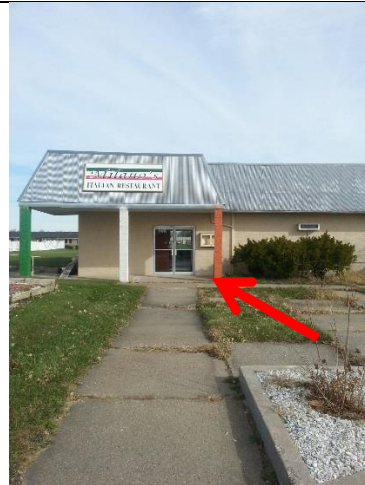
Photo 4: View of building entrance and west side.
